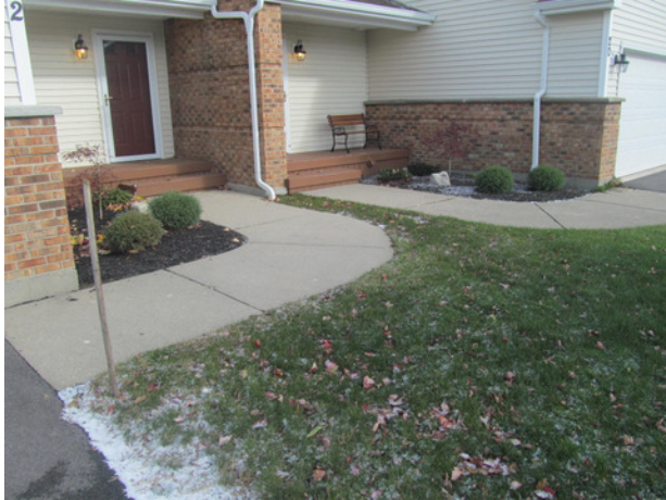
Concrete sidewalk overview
