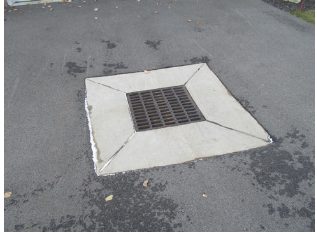
Typical catch basin at asphalt pavement
