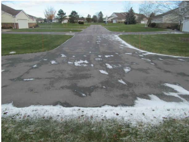
Asphalt access drive overview
