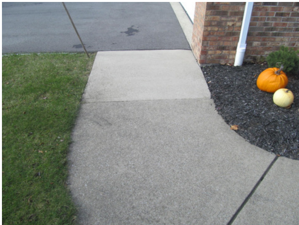
Previous partial concrete sidewalk replacement near Building 29
