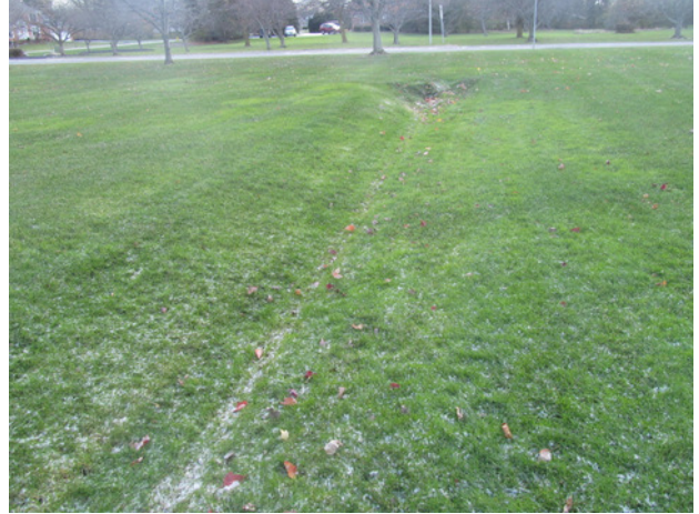
Drainage swale overview (near the community's entrance)
