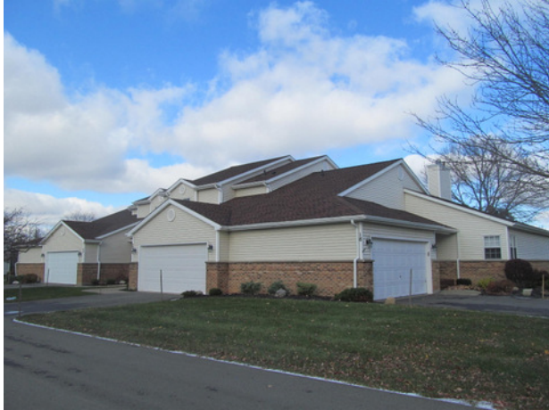
Asphalt shingle roof overview at Building 2
