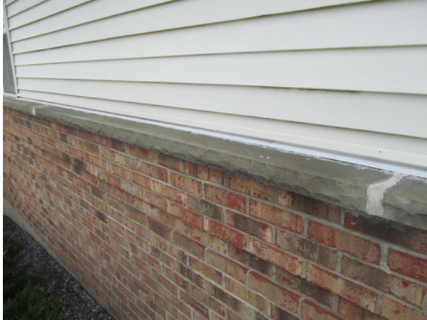
Masonry wall overview (note masonry sill)
