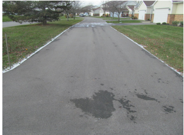
Asphalt access drive overview
