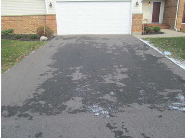
Asphalt driveway overview
