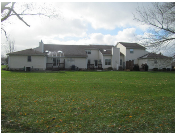
Typical rear elevation of three-unit building
