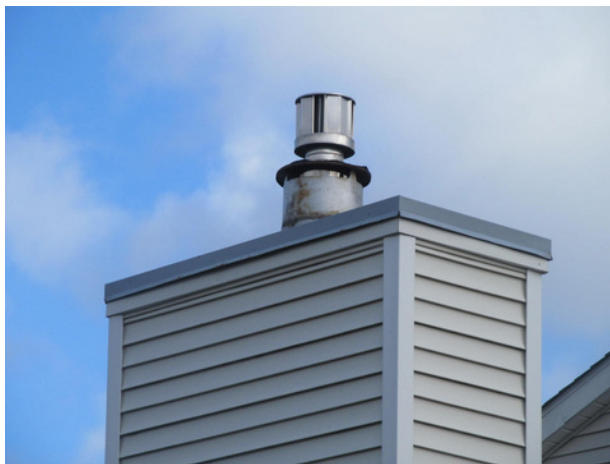
Typical metal chimney cap
