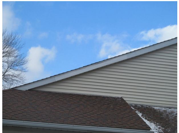
Previous partial fascia cladding replacement at Building 17
