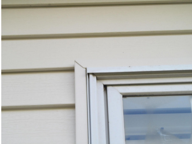
Typical J-channel and vinyl siding/window interface
