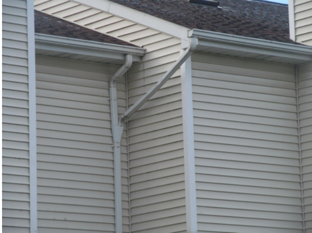
Aluminum gutter and downspout overview
