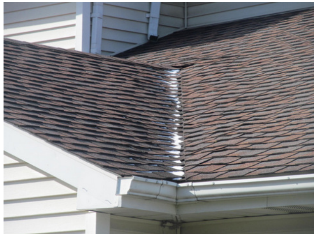
Typical enclosed half weaved valley at asphalt shingle roof
