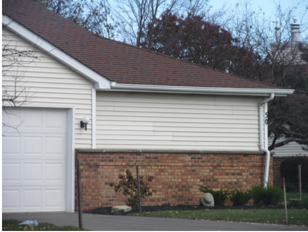
Previous partial vinyl siding replacement at Building 5
