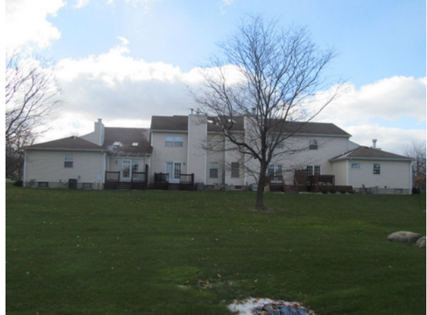
Typical rear elevation of four-unit building
