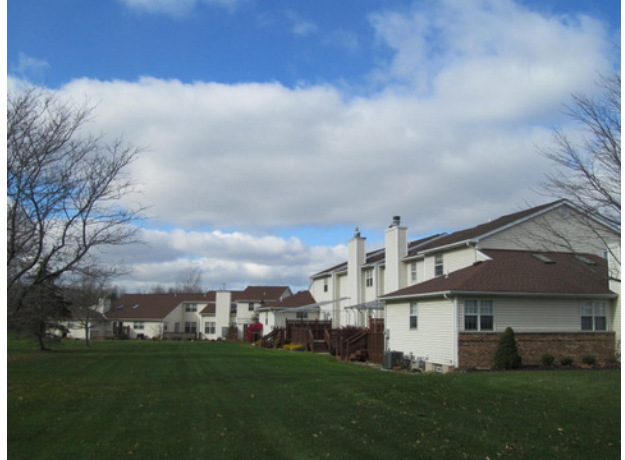
Asphalt shingle roof overview at remaining buildings
