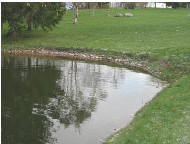
Isolated shoreline erosion and deterioration along east portion of pond shoreline
